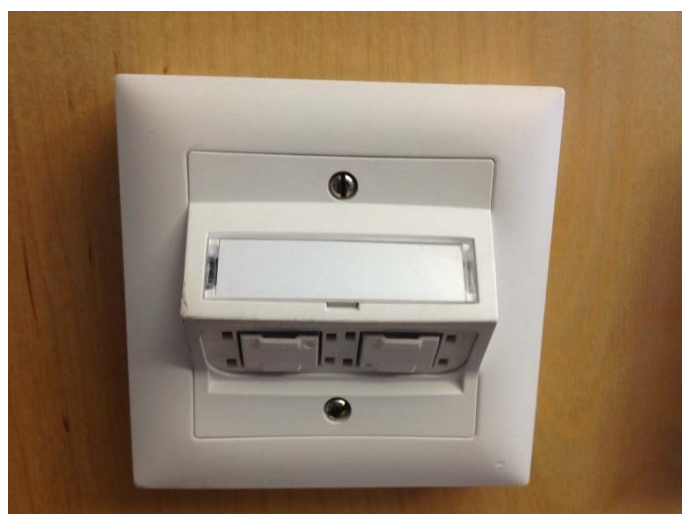
Figure A.1: Example of Integrated Wall Plug
