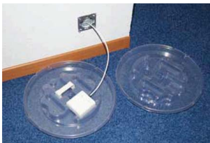
Figure E.1: Optical fibre home cabling system
