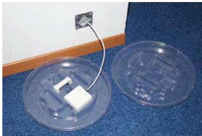
Figure E.1: Optical fibre home cabling system
