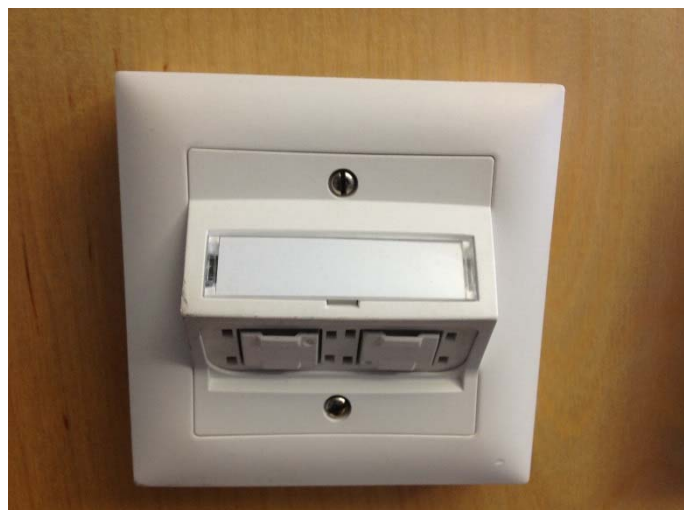
Figure A.1: Example of Integrated Wall Plug
