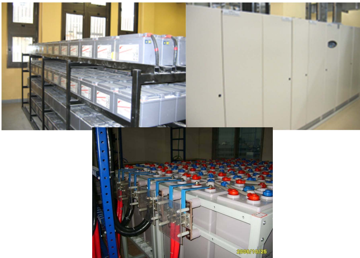
Figure A.3: UPS multi-string batteries on shelves or in cabinets
