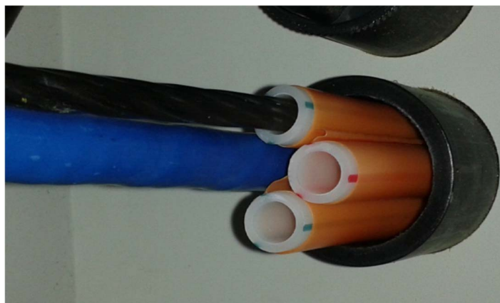
Figure 9: Installation of sub-ducts to provide segregation
