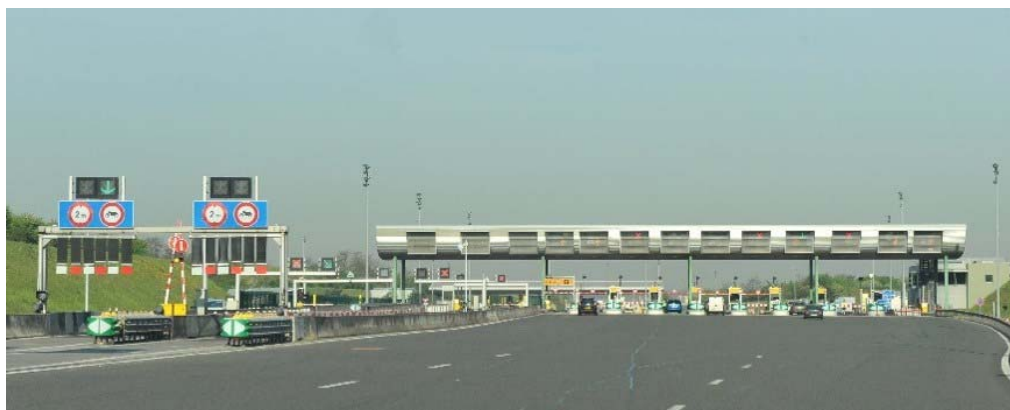
Figure 20: Toll plaza with non-stop ETC lanes (left), stop&go ETC and automatic lanes (right) (ETSI TR 103 579 [i.8])
