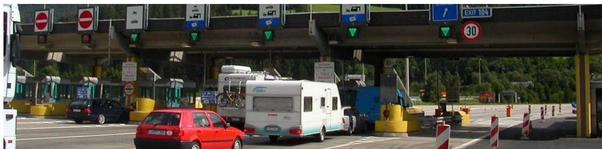
Figure 19: Toll plaza with non-stop ETC lane (far left), stop&go ETC (centre lanes) and automatic lane (right) (ETSI TR 103 579 [i.8])
